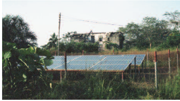
The solar panels in the hospital grounds that provide electricity for the wards and the lab
