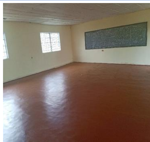
Refurbished learning space
